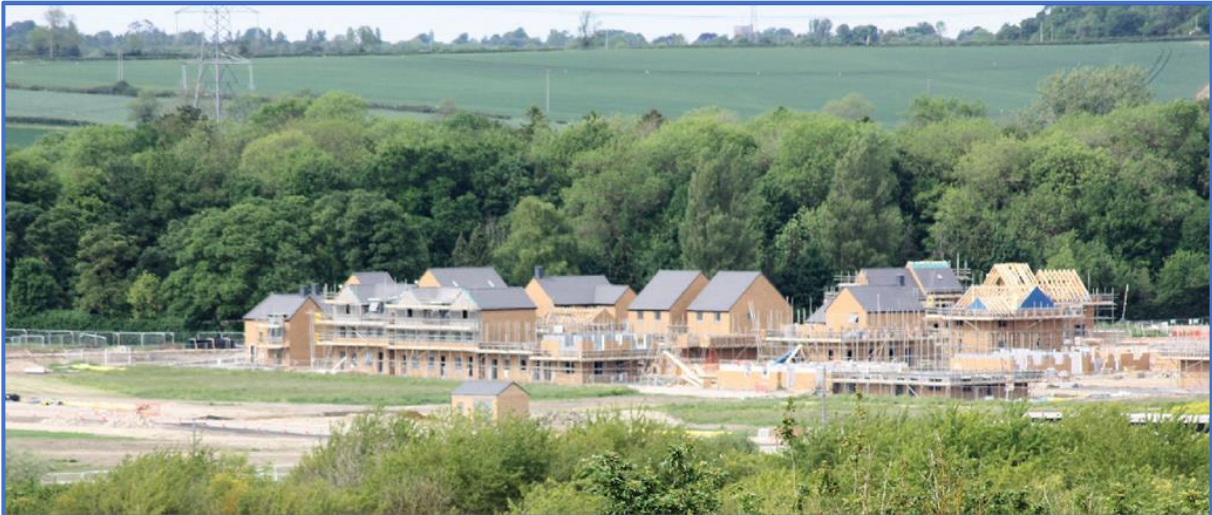
Figure 2: New housing being built in Bidwell West
